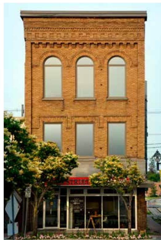
This 1890’s triple brick building at 40 King Street in Waterloo was gutted and retrofitted to achieve a 70% energy use reduction.
